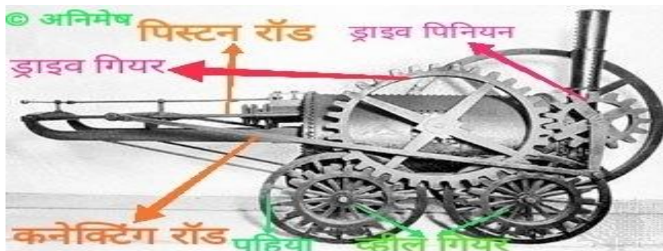
1 st Steam locomotive by Richard Trevithick Speed 15 Mph
