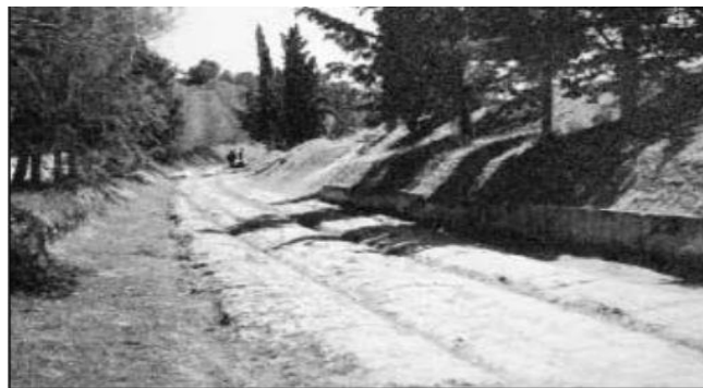
About 1.1 Km length of Rutway found
